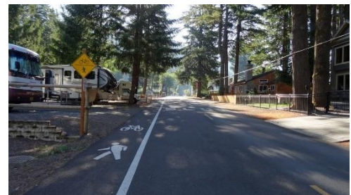
Image 16 – Visually separated pedway on a rural road.
